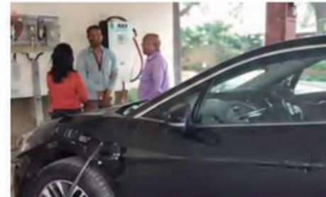
EV Charger installation in India
