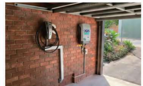
EV Charger Installation in Sydney Australia
