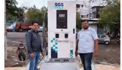
EV Charger installation in India
